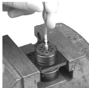
6. Secure connector in a smooth jaw vise and place contact in appropriate cavity of receptacle.
