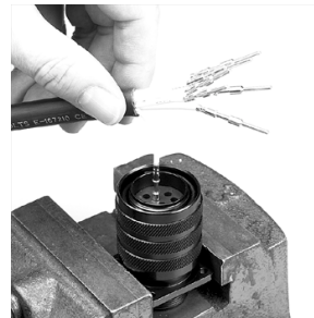
11. Place contact in appropriate cavity of plug. (properly lubricate - refer to step 5)
