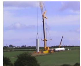
Lower Tower Erection
