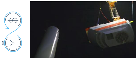
Nacelle Installation
