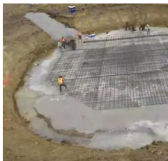
Turbine foundation Reinforcement
