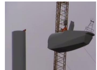
Nacelle Installation
