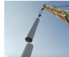
Upper Tower Erection
