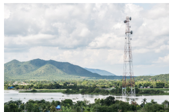
WIRELESS / BROADBAND / DATA CENTER Pg. 140
