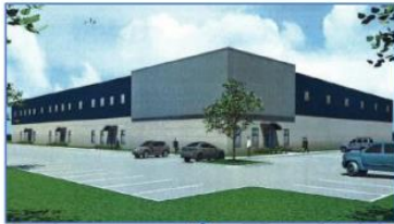
New Warehouse & Light Assembly Facility Milton, WI 60,000 sq. ft.
